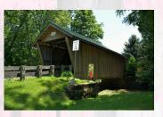
The bridge, which spans the Sunday Creek, was built in 1875, closed in the late 1980s, and repaired in 1994. Major repairs were made in 1994, including steel piers and new siding and roof. The bridge was listed on the National Register of Historic Places in 1999.
