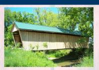
The bridge was built in 1872 and at a length of 84 feet, it crosses Wolf Creek. The bridge was built for \$729.96. Because of flood problems, the bridge is anchored with steel beams to its abutments. The road to the bridge is closed to all but pedestrian traffic.
