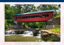
The bridge was built for \$872.00 and is 74 feet long crossing Island Run. A center pier was added in the 1940s, then in the 1950s, the center pier was replaced. In 2008 the bridge was redesigned and rebuilt and a Burr arch was added. The center pier was removed during the 2008 redesign.
